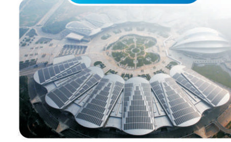
Xincheng International Expo Center 10 MW Photovoltaic Power Generation Project
