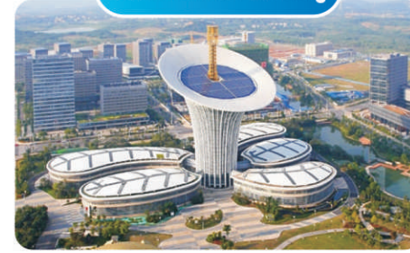
Future Science & Technology City Photovoltaic Grid-connected Power Generation Project
