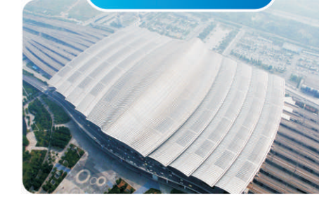
Wuhan Railway Station 2.2 MW Photovoltaic Power Generation Project
